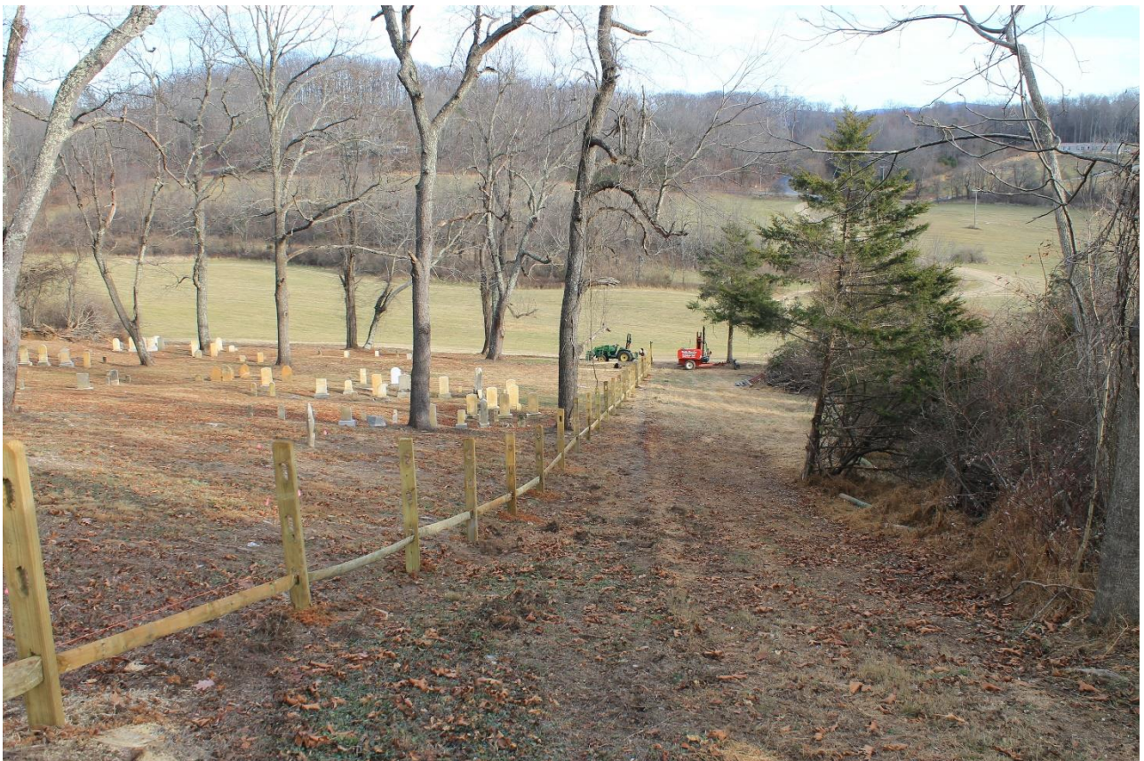
Because of the steep terrain, all of the work had to be done from top to bottom.
