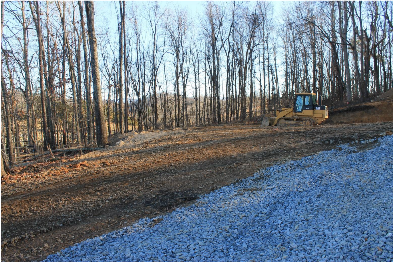
The new site for the schoolhouse. Only 100 ft. or so from its original location.
