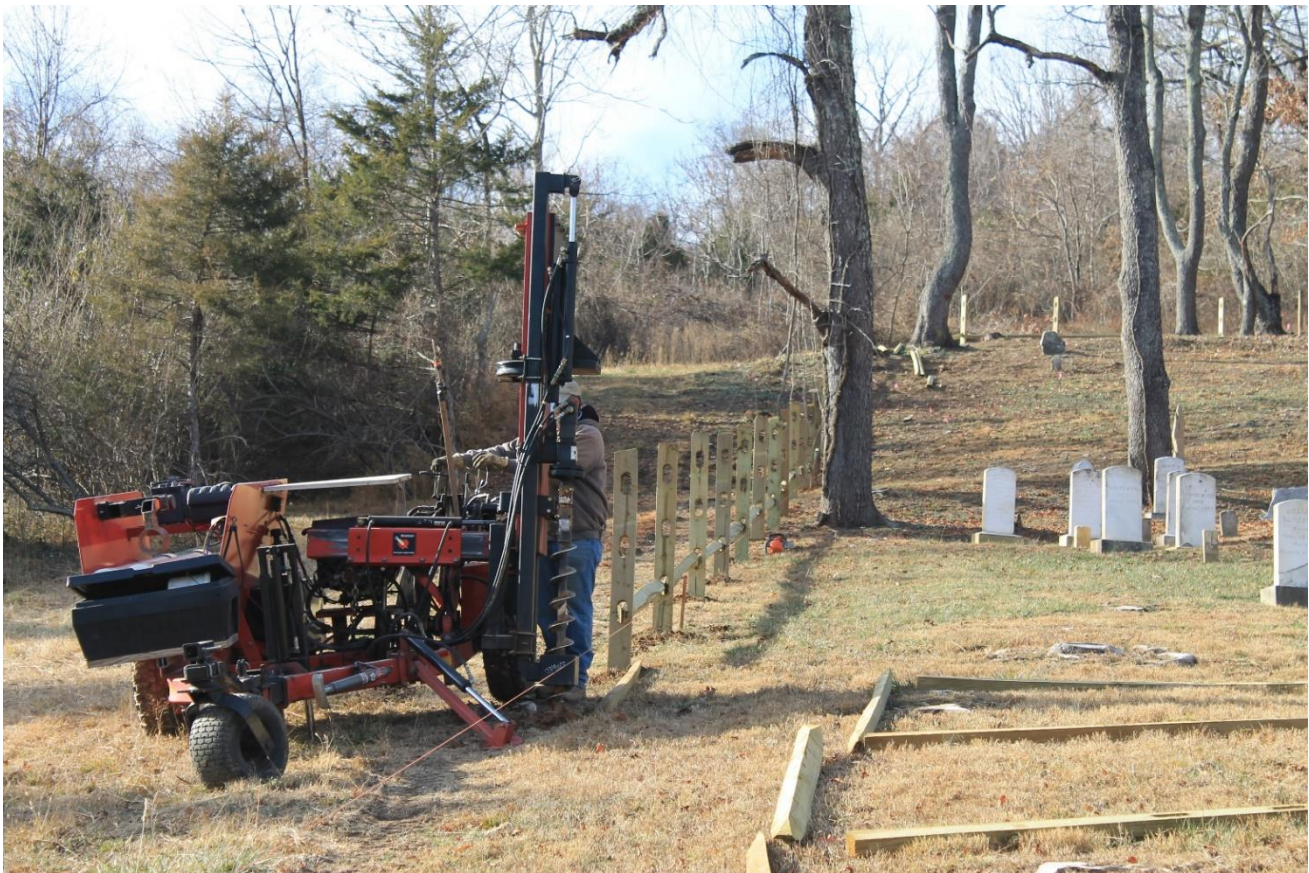
Getting started-The old barbed wire fence and posts have been removed and the new posts and first rails are going in!
