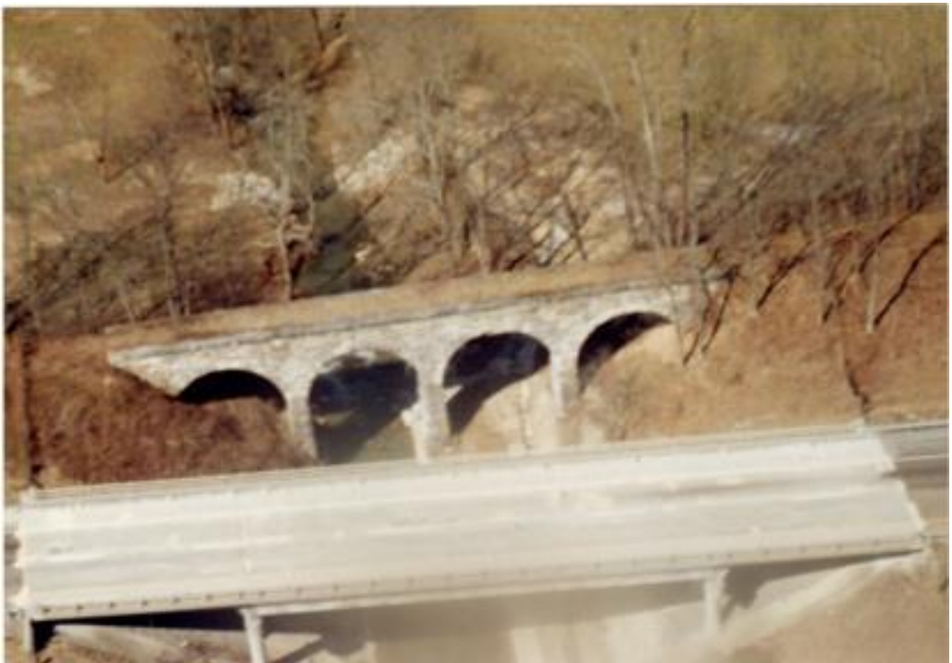
Valley Railroad (B&O) Stone Trestle at Mint Spring, Virginia
