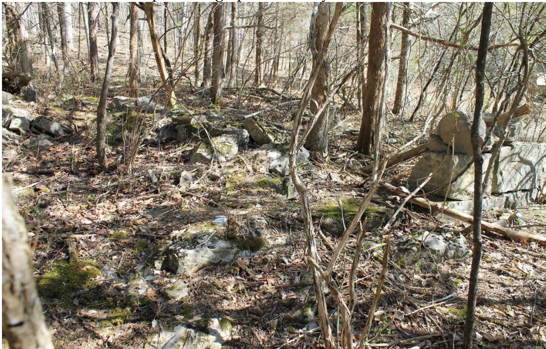
Above: The foundation was constructed of exceptionally large hand cut stones that seem to have fit together so perfectly that they appear to have been dry stacked with no mortar needed.
