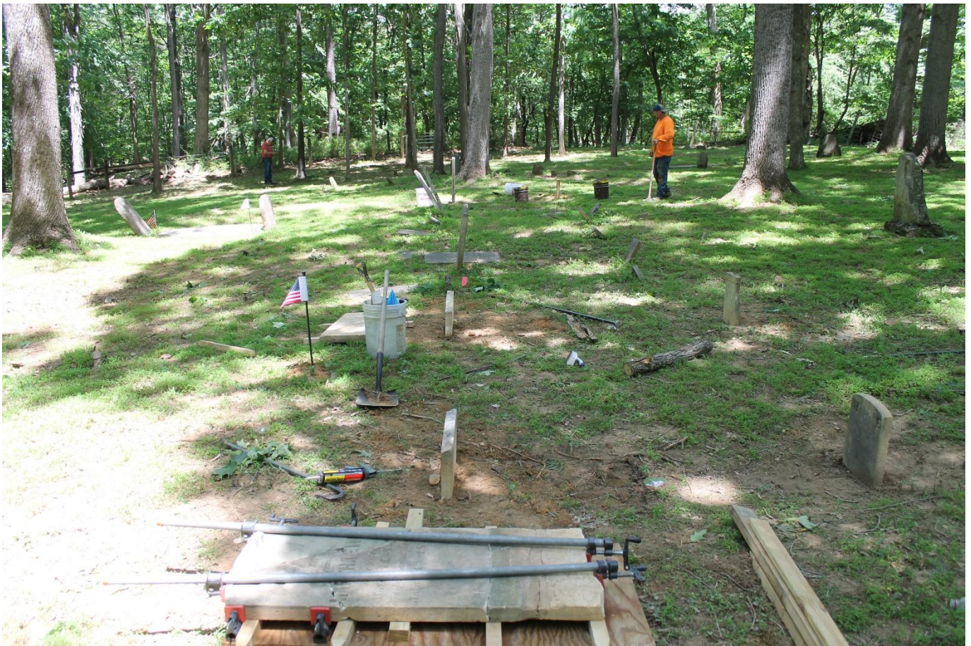
The stone on the platform being clamped was broken in five pieces. Soon to be reset in one piece.
